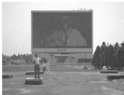
3D camera and lenticular photo inventor Allen Lo in front of the giant Sony Jumbotron at Expo 85 in Japan. Made of thousands of very bright CRT's, it was later covered with strips of polarizer & used to project 3D video.
